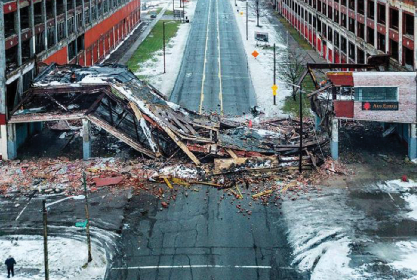
The bridge as it looked on the morning of January 24, 2019
